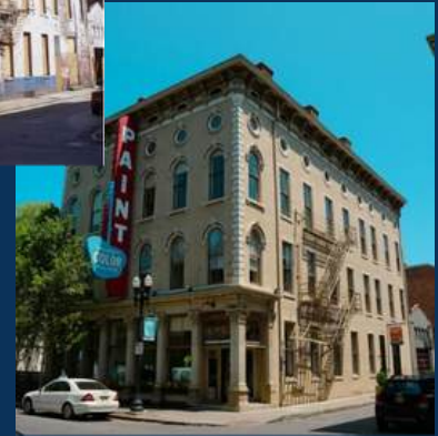
After 3CDC redevelopment
