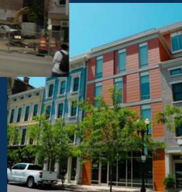
After 3CDC redevelopment
